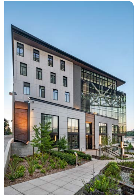
Achieving the delicate balance of solar heat gain protection, optimizing daylighting and providing views, Weber Thompson specified Solarban ® 60 glass for the storefront and punched openings for Watershed.
