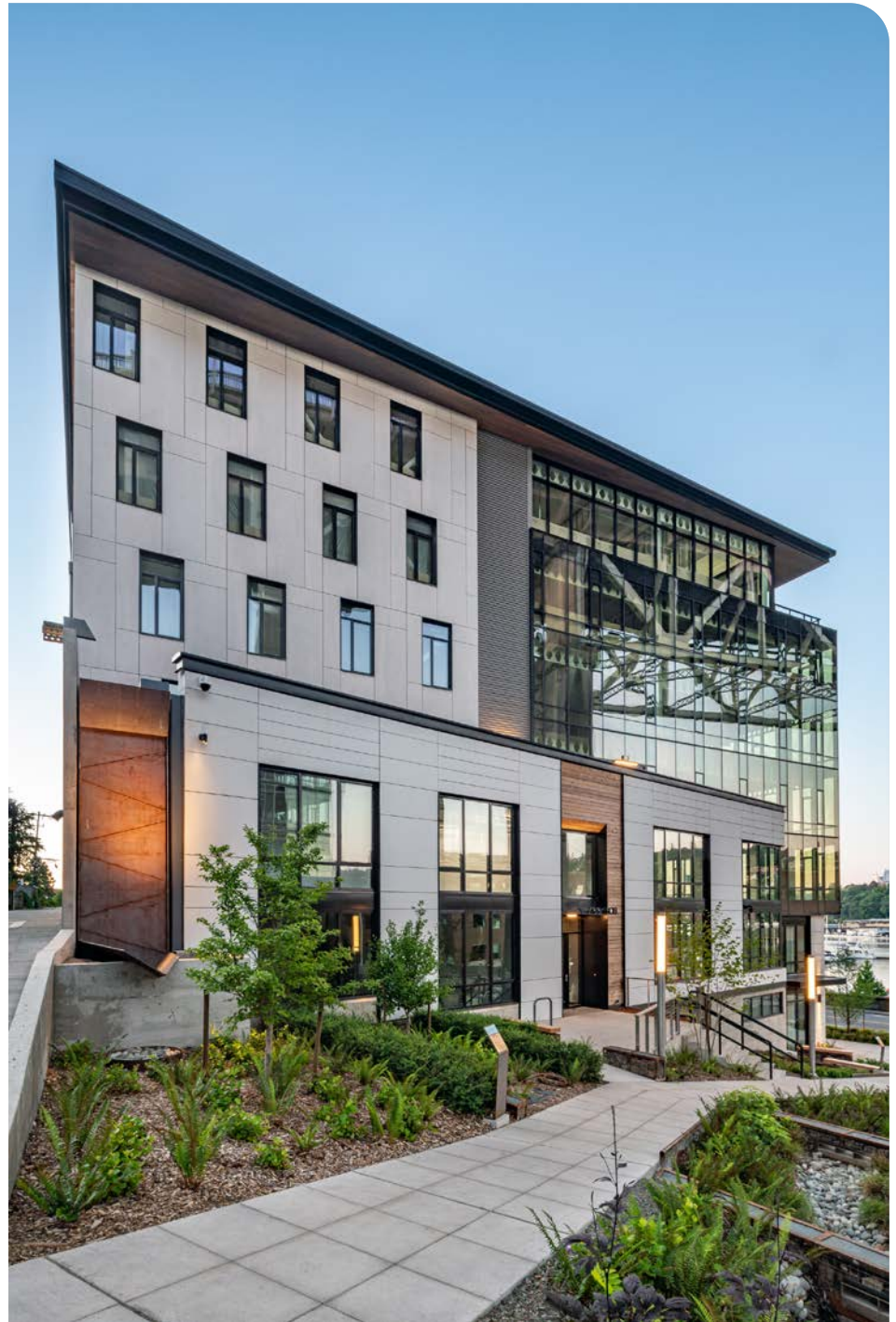
Solarban® 60 glass by Vitro Architectural Glass contributes to 7-story Watershed's Living Building Challenge petal certification and to meeting Seattle's Living Building Pilot Program's stringent requirements, which include using 25% less energy per square foot than a baseline office building.
