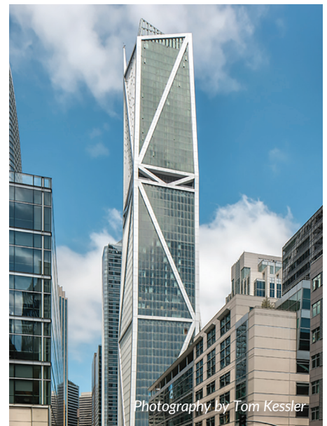
The angled design of 181 Fremont disrupts airflow to minimize wind load and reduce stress on the glass and frames.
