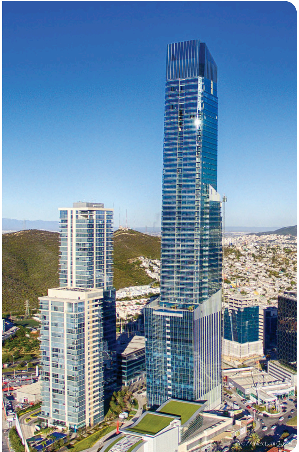
Rising majestically in the shadows of the Sierra Madre range, Koi Sky Residences, glazed with Solarban® R100 glass on tinted Optiblu® glass, cuts a dramatic figure in “The City of the Mountains.”
