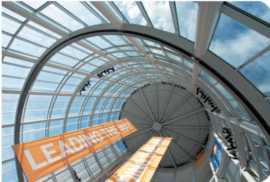
*Solarban*® 60 glass by Vitro Architectural Glass transmits light into Prudential Center through two 110-foot-tall glass and steel cylinders.
